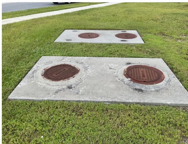
Storm water control structure
