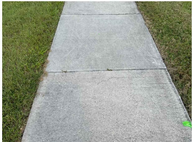
Sidewalk cracks
