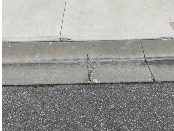
Concrete spalls
